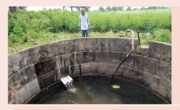
Well recharge is a simple low-cost technique to recharge the ground water which in turn increased the cropping intensity and productivity.
